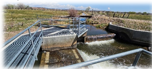
Lake Fork Connector Pipeline Heading April 22, 2024
